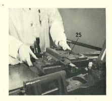
9. Place the matrix heads base (25) on the main stand, locating the keys in the keyways. Release the locating key distance piece clamp screw and place the distance piece in the required point size position. Tighten the clamp screw.
