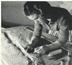
ABOVE: Making a hillshading model with plasticine for photographing on a process camera.
