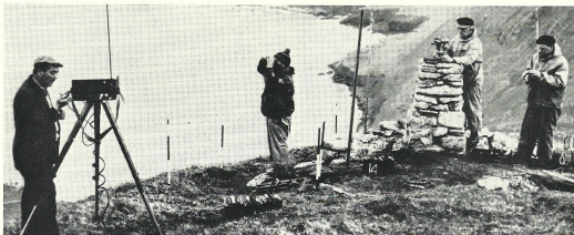
ABOVE Triangulation party on St. Kilda. In areas of outstanding natural beauty the triangulation pillars are built in local stone as shown in this photograph.
