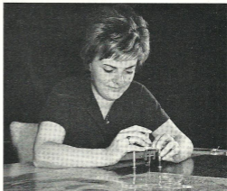
ABOVE Scribing map detail on glass with a circle cutter.
