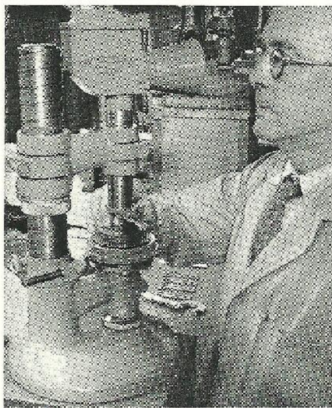
Fig. 13: Experienced operator using measuring comparator to detect errors down to a quarter of one ten-thousandth part of an inch during blade manufacture
