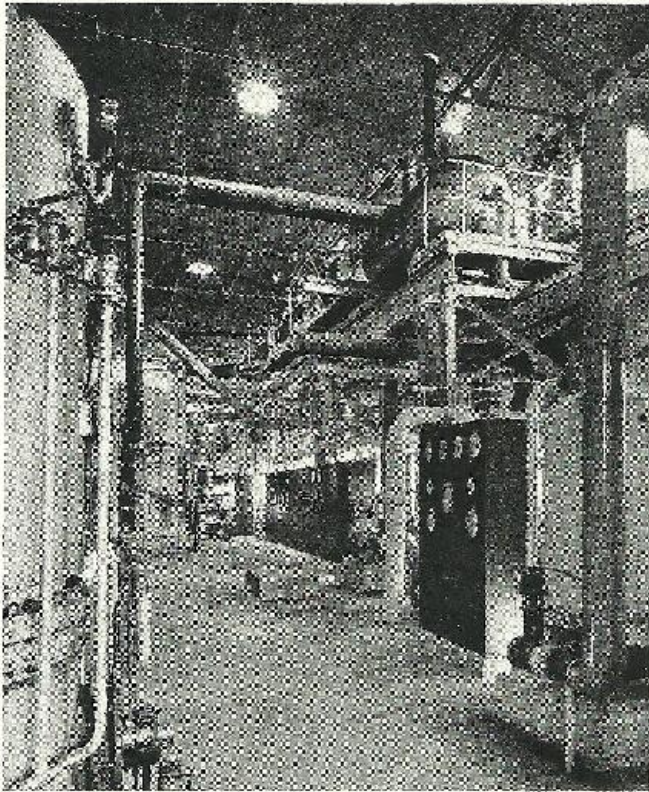
Fig. 2: Part of the new Power House
