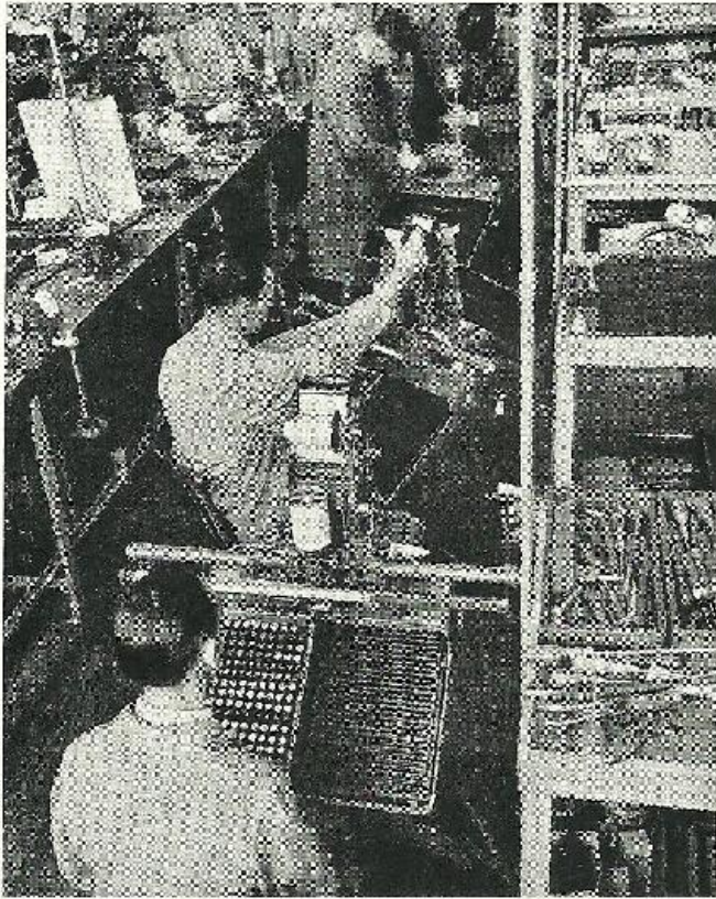
Fig. 21: Progressive final assembly of keyboards
