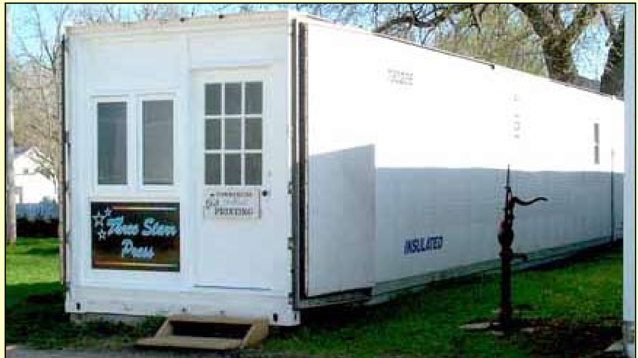
Here's the shop showing the walk-in door and two opening windows. I left the heavy doors on, so I can lock it up securely.
